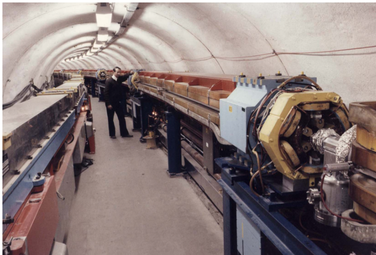
Figure 2.2: Picture taken in the tunnel, with synchrotron on the left and storage ring on the right
